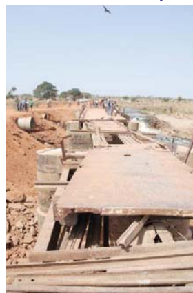
Eloki Bridge on the Wau-Aweil Road, 24/01/08 Finne Lucey, UNJLC Logistics Officer
