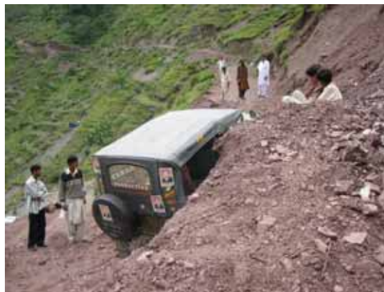
A Jeep trying to negotiate a road where landslides have occurred recently. Photo: UNJLC.
