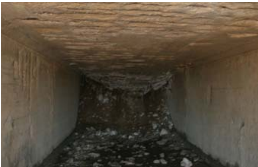
Underneath Arrida Bridge
