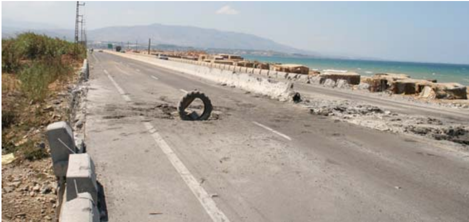
Approach El Aadbe Bridge
