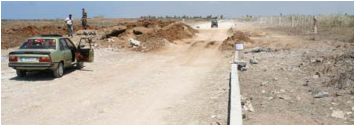
Approach Arrida Bridge
