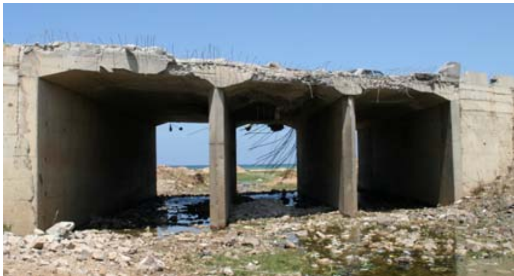
Underneath El Aadbe Bridge
