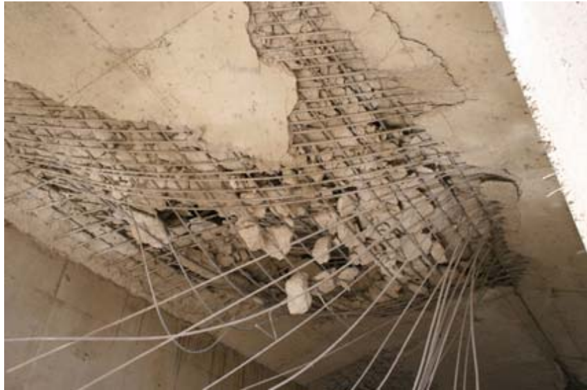
Underneath El Aadbe Bridge
